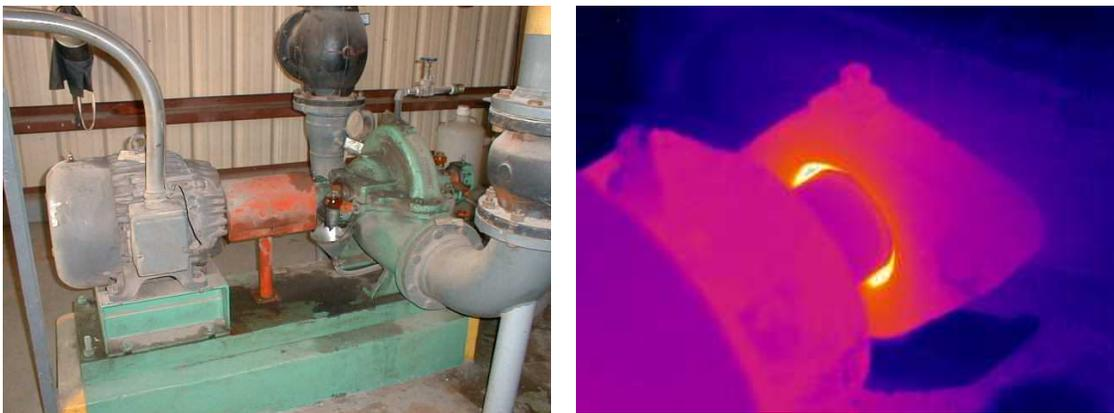
*Figure 6. Visual and thermal images of a cooling water pump*
